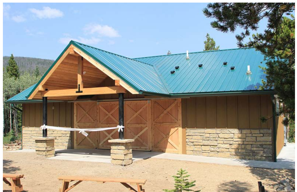
The completed shower house during the dedication.
